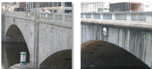
Glass recycled from Temple University was used in the recent restoration of the Market Street Bridge of Philadelphia, PA.
